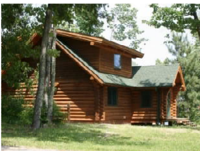
Rear of Cabin
