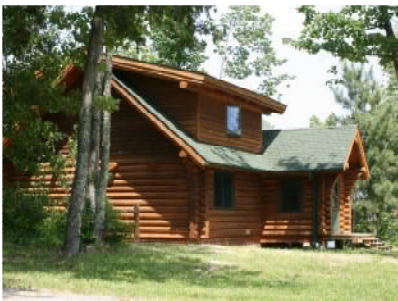
Rear of Cabin
